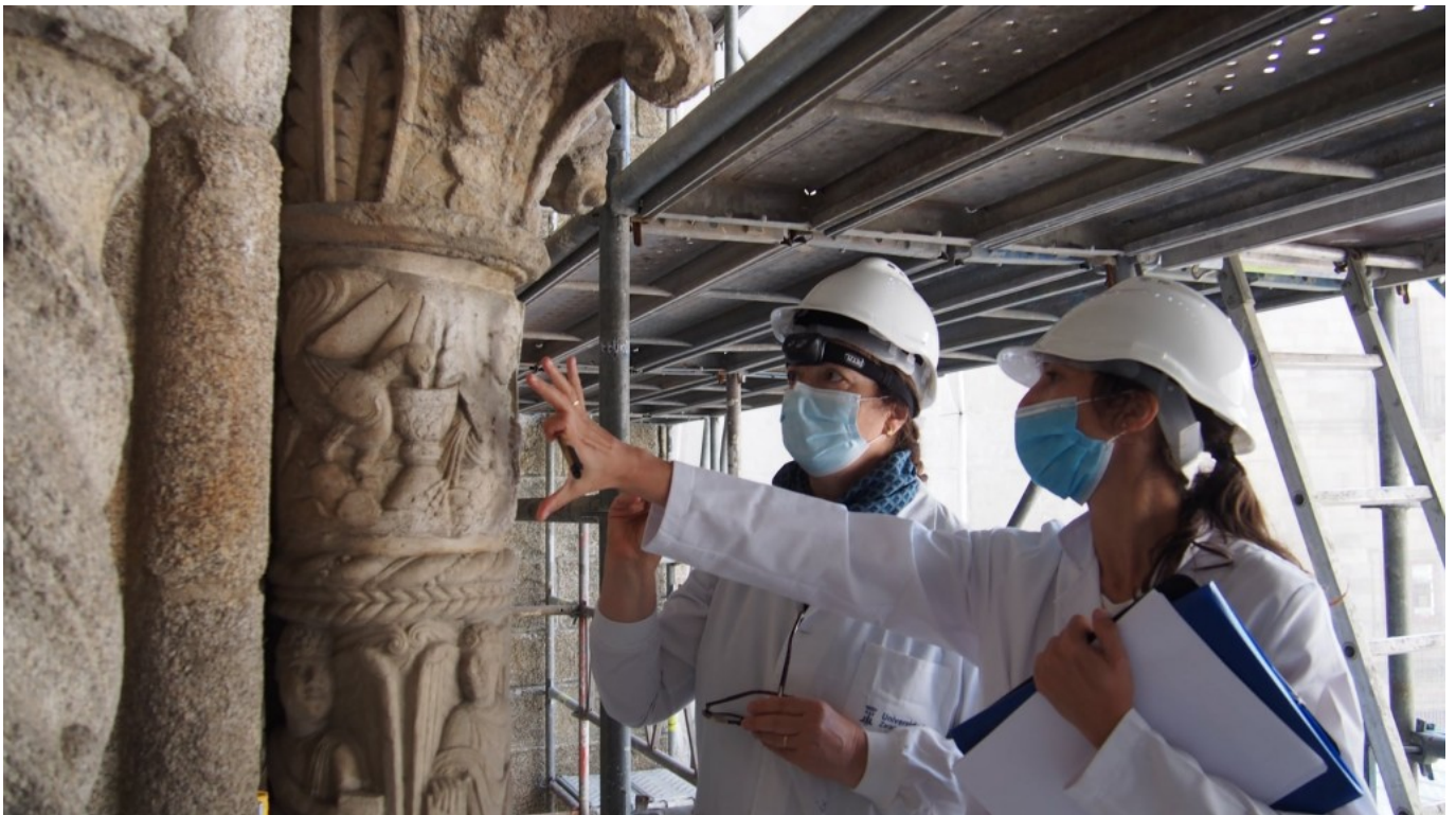
Pilar Lapuente and Silvia González examine one of the marble columns of the Chatedral of Santiago de Compostela. Photo: ICAC (CC BY-SA 4.0).
