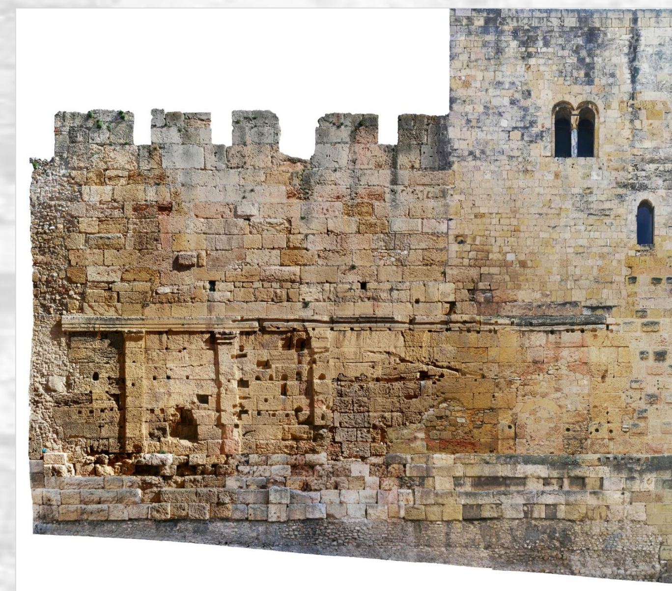
Ortho-image of wall facing of the "Torre del Pretorio"
